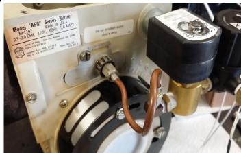
25. Install the retention head. It just slips onto the blast tube. If the head is too loose, you can kink the band a bit to make it fit more snugly on the blast tube. **The nozzle should be flush with the inside of the head to 1/4" behind the head.** (you can bend the head in or out some if necessary). Make sure the nozzle is centered in the retention head. Sometimes you need to gently force the preheater to one side or another.
