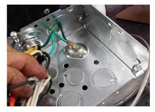
29. Wire burner according to wiring schematic.
